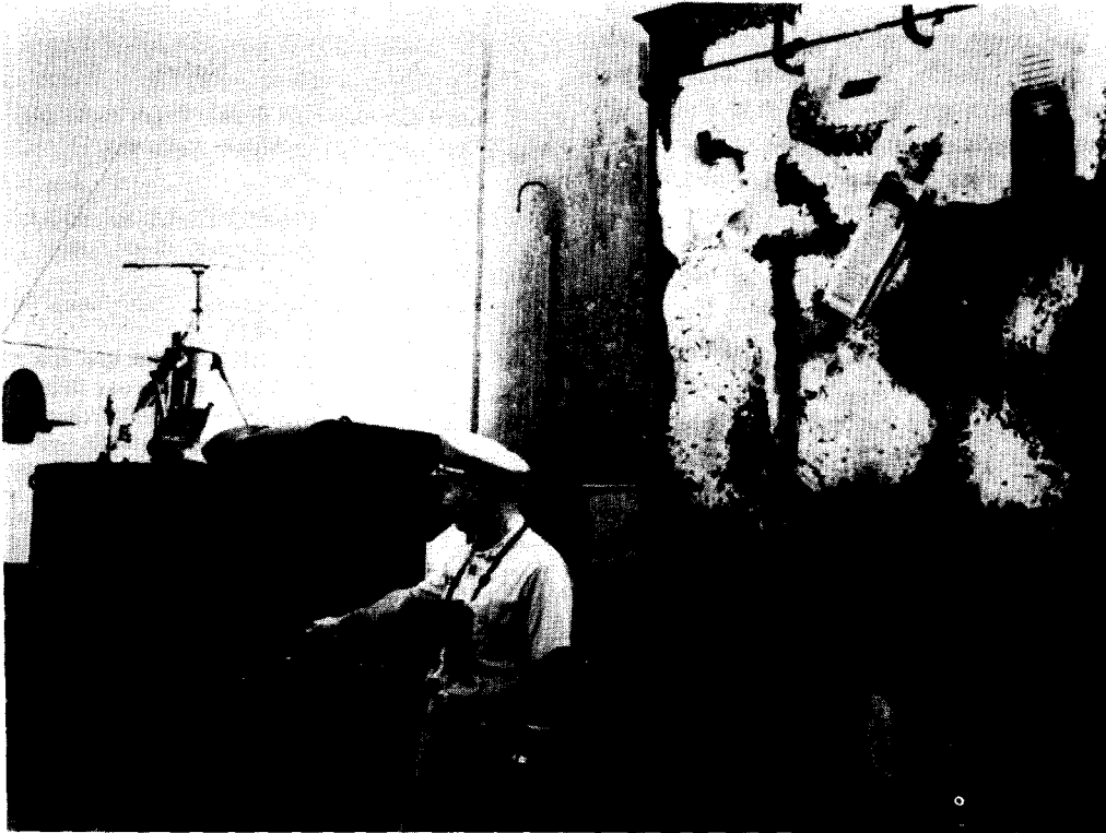
(U) The Captain of the Liberty , CDR William L. McGonagle, surveys the damage done below the bridge from the rockets fired by the Israeli aircraft.
