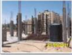
Expansion of 8 existing schools
