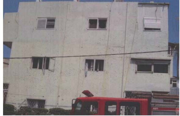
A building 30 yards from the site of impact damaged by ball bearings
