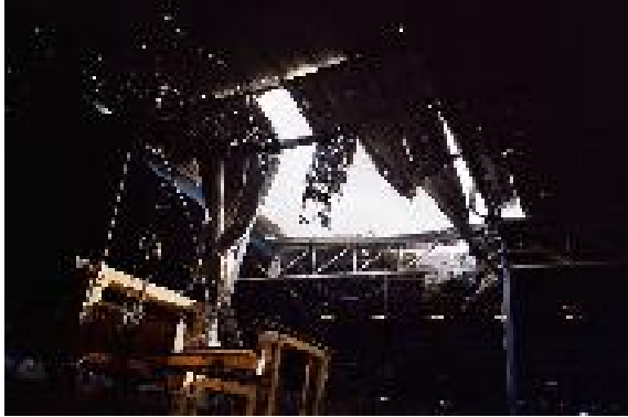
A hole in the roof of a factory located in northern Israel. The industrial zones in the north were a Hezbollah target, as shown by the seized range cards (see Appendix 5ii).
