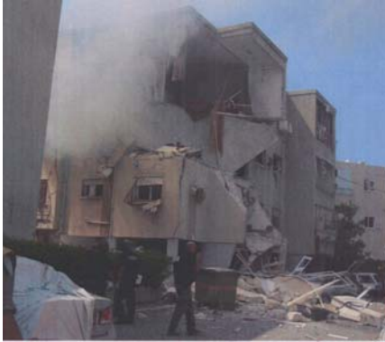
The collapse of the front of the building
